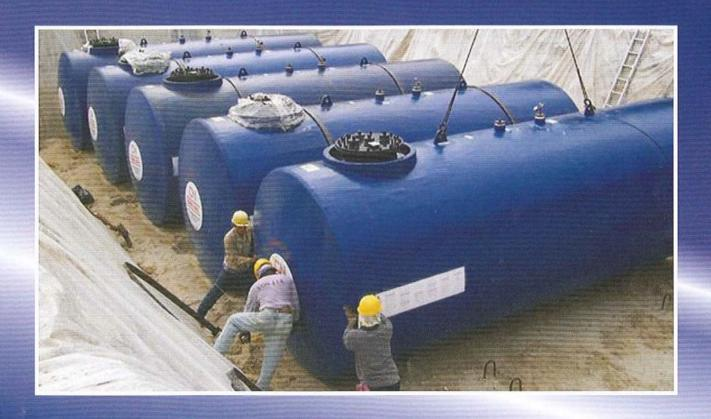
An environmentally safe double-wall, corrosion-resistant secondary containment with the strength of steel
