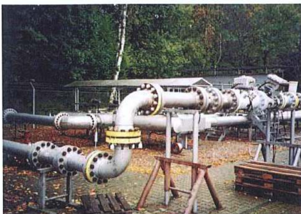
Research at HP test rig Lintorf (Germany)
